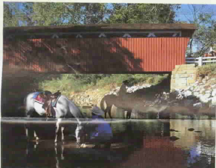
A refreshing break under the Everett Road covered bridge.
